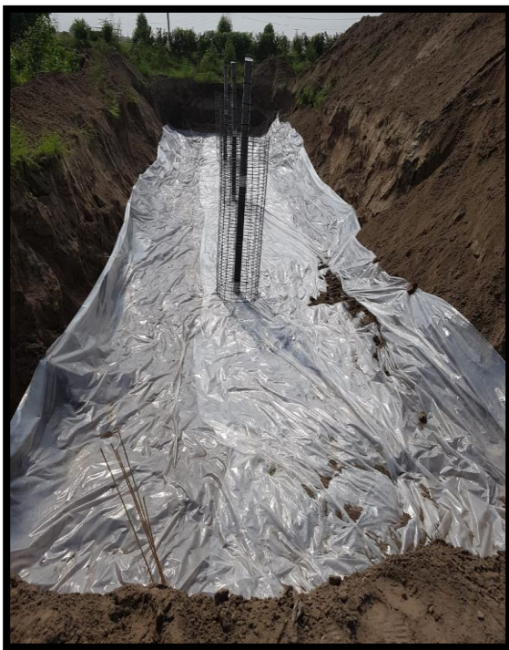
Installation of Gas Vents
